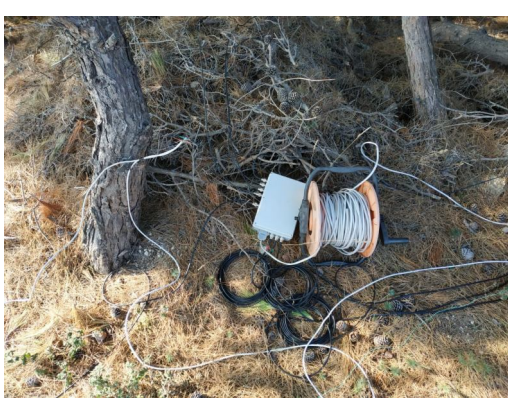
RX antennas switch
